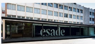
Building 1 - Av. Pedralbes
